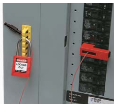
3. Pass plastic key through lock rail and attach lock, preventing key from sliding down cable and opening lockout device.
