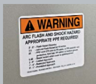
Arc Flash Labeling
